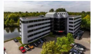
Refurbishment value chain at B-Right (Amersfoort, Netherlands)
