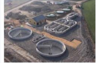
Infrastructure Replication, Waste Water Treatment Plant (Spain)
